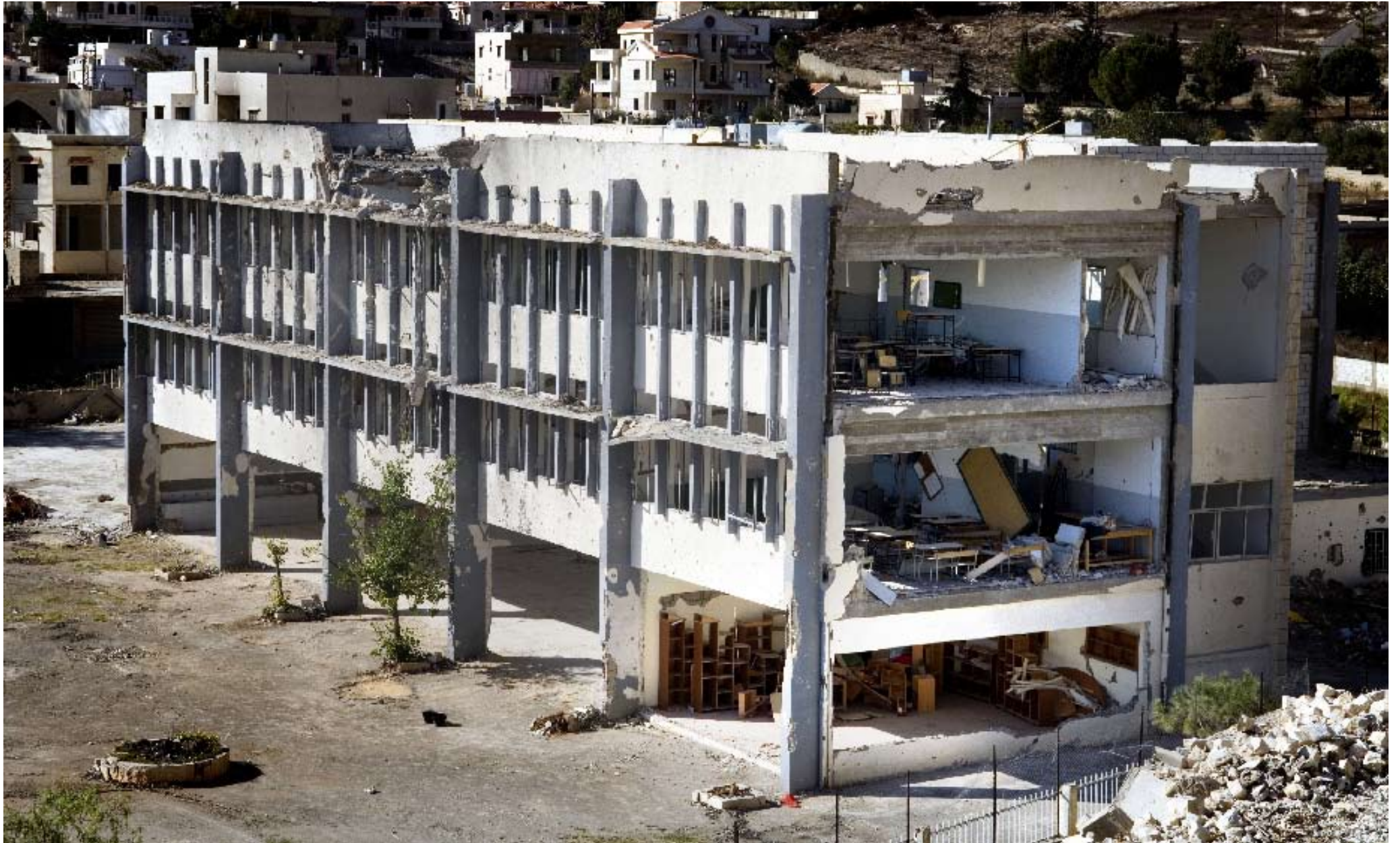
Repairing Lebanon (school) 2007 50 x 30 cm
